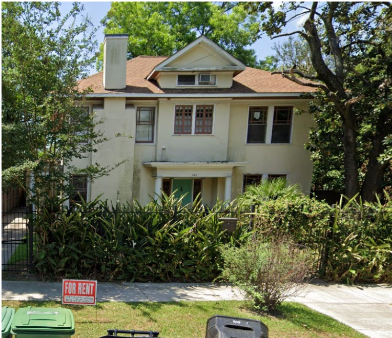
Figure 1 - 509 Sul Ross, next door neighbor.
